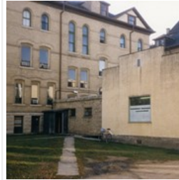
Clark Hall - west side
