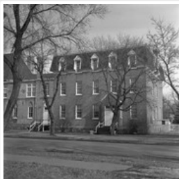
St. Augustine's Roman Catholic Church Offices
