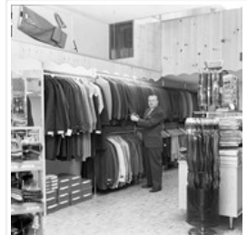
Watt's Men's Wear - interior
