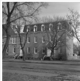
St. Augustine's Roman Catholic Church Offices
