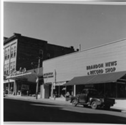
100-block 10th Street, facing southwest
