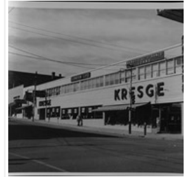
Southwest corner 10th Street and Rosser Avenue
