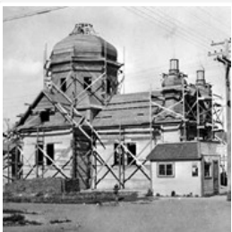
Construction of St. Mary's Ukrainian Catholic Church
