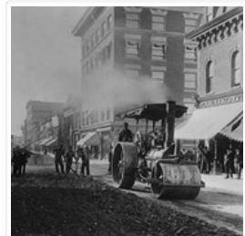
Paving Rosser Avenue
