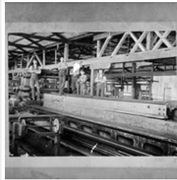
Interior of Hanbury Mill
