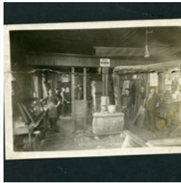
Hanbury Manufacturing Co. - Sash and Door Department
