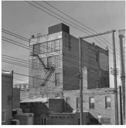
Former Christie Building - From Rear
