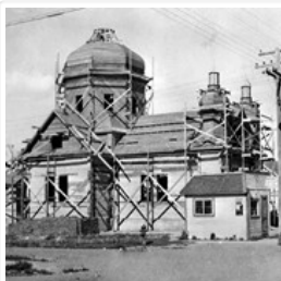
Construction of St. Mary's Ukrainian Catholic Church
