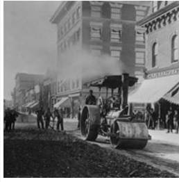
Paving Rosser Avenue
