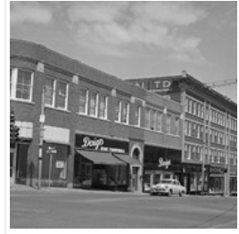
10th Street Businesses - West Side of 100 ...
