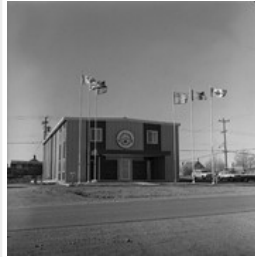
Dakota-Ojibway Tribal Council Building
