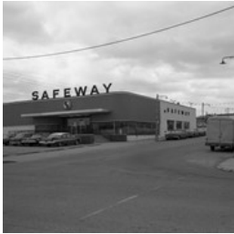
Safeway - Princess Avenue and 6th Street
