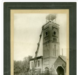
Original Fire Hall
