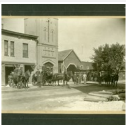
Original Fire Hall
