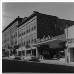
100-block 10th Street, facing southwest (2)
