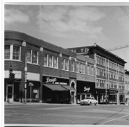
West side of 10th Street from Princess Avenue, ...
