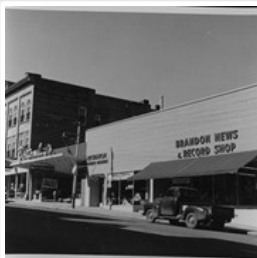
100-block 10th Street, facing southwest
