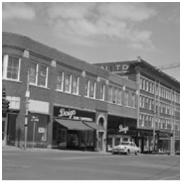
10th Street Businesses - West Side of 100 ...
