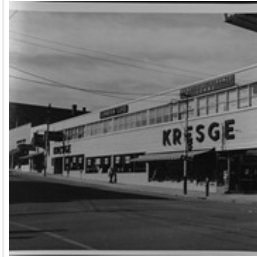
Southwest corner 10th Street and Rosser Avenue
