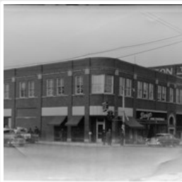
Hughes Building, Brandon, Manitoba
