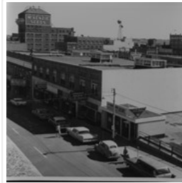
East side 10th Street facing north from Princess Avenue, Brandon, ...
