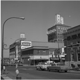
000 and 100 Blocks of Tenth Street
