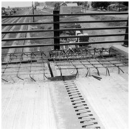
Construction of third First Street bridge
