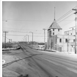
Second First Street bridge
