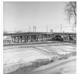
Second First Street bridge
