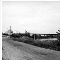
Construction of third First Street bridge
