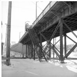
Second First Street bridge
