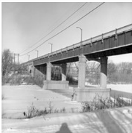
Second First Street bridge
