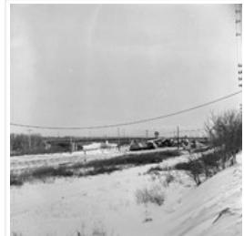
Second First Street bridge
