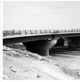
Construction of third First Street bridge
