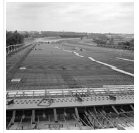
Construction of third First Street bridge
