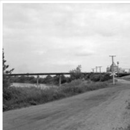
Construction of third First Street bridge
