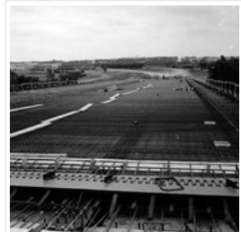
Construction of third First Street bridge
