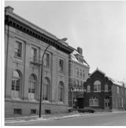
Merchants Bank of Canada Buildings
