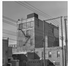
Former Christie Building - From Rear
