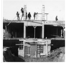
A.E. McKenzie Building construction
