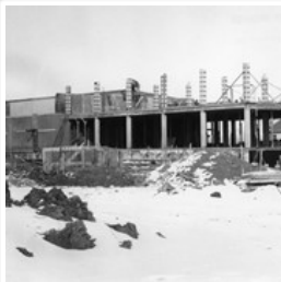
A.E. McKenzie Building construction
