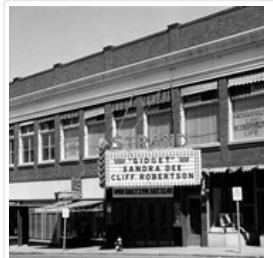
Hughes Block (Strand Theatre building)
