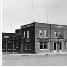
Gillis & Warren Building
