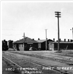
CNR Engine Terminal
