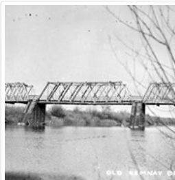
Assiniboine River Bridge North of Kemnay
