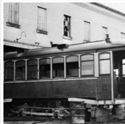
Dismantling of Streetcar No. 8
