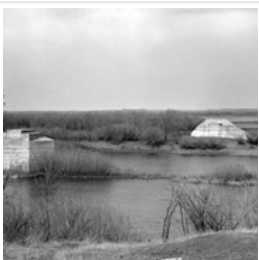
Grand Trunk Pacific Bridge Piers
