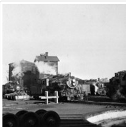
CNR Engine Terminal
