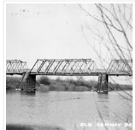
Assiniboine River Bridge North of Kemnay
