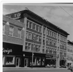
West side of 10th Street facing north from ...
