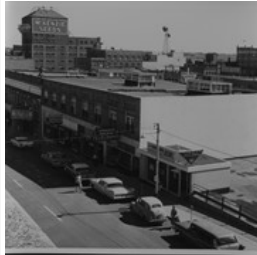
East side 10th Street facing north from Princess ...
