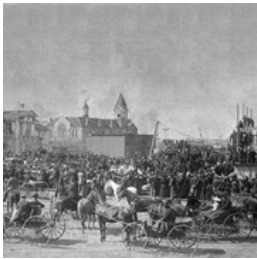
Methodist Church Under Construction
