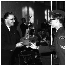
Air Force inspection
