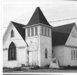
Former Church, now Community Hall, Chater, Manitoba.
