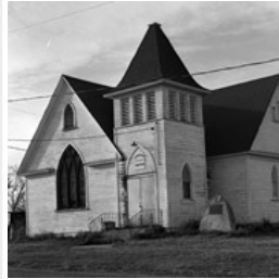
Former Church, now Community Hall, Chater, Manitoba.
