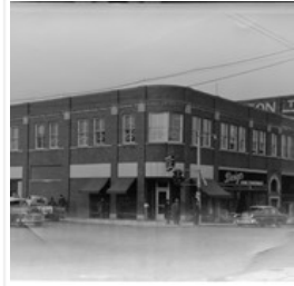
Hughes Building, Brandon, Manitoba
