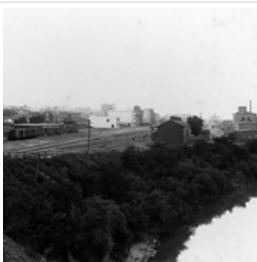
View from 1st street bridge looking west
