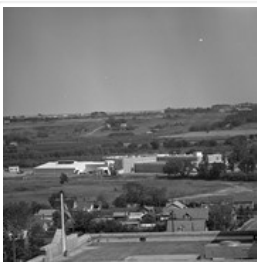
Brandon from roof of Christie Building
