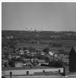
Brandon from roof of Christie Building
