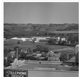
Brandon from roof of Christie Building
