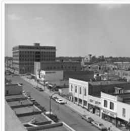
Brandon from roof of Christie Building
