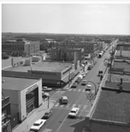
Brandon from roof of Christie Building
