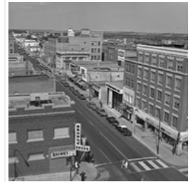
Brandon from roof of Christie Building
