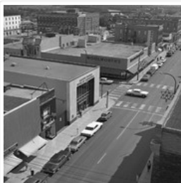
Brandon from roof of Christie Building
