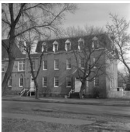
St. Augustine's Roman Catholic Church Offices
