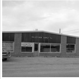
Valleyview Supply Co.
