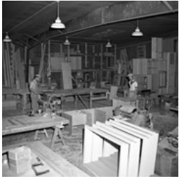
Valleyview Supply Co.
