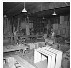
Valleyview Supply Co.
