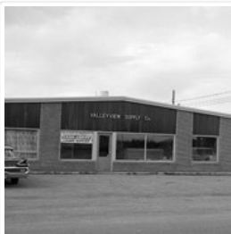
Valleyview Supply Co.
