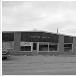
Valleyview Supply Co.
