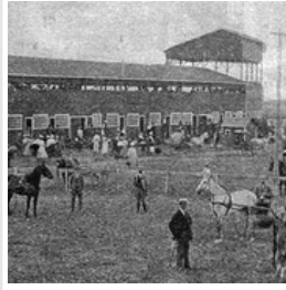
Fairgrounds in Rear of Original Grandstand
