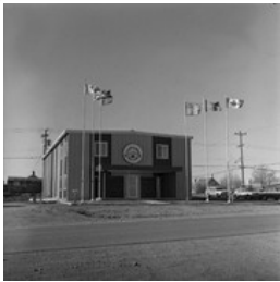
Dakota-Ojibway Tribal Council Building
