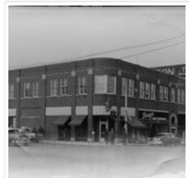
Hughes Building, Brandon, Manitoba
