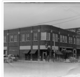
Hughes Building, Brandon, Manitoba
