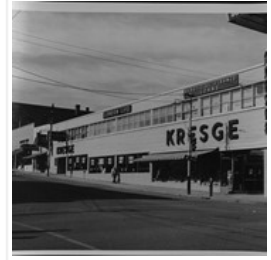
Southwest corner 10th Street and Rosser Avenue
