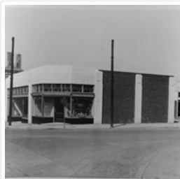
Northeast corner of 10th Street and Princess Avenue, ...
