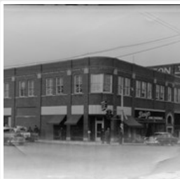
Hughes Building, Brandon, Manitoba
