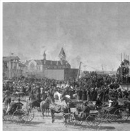
Methodist Church Under Construction
